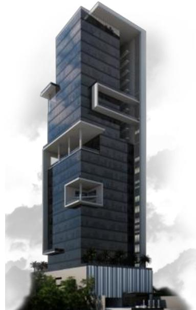
The selected materials are of the highest quality, which include, granite and marble floors and walls. Thinking about energy consumption and maintenance costs reduction, double tempered Low-e glass facade was contemplated in the west facade, which generates an air of 6mm which helps decrease by 20% the thermal load of the building by the action of the sun, resulting in significant energy savings.
